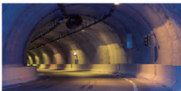
Self-Localization within Tunnels
